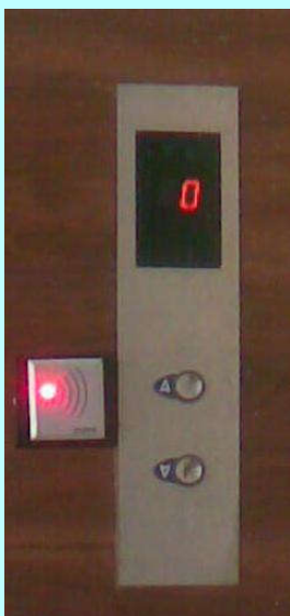
Elevator with Access Control. Only Authorized Card Holders can use the elevator
